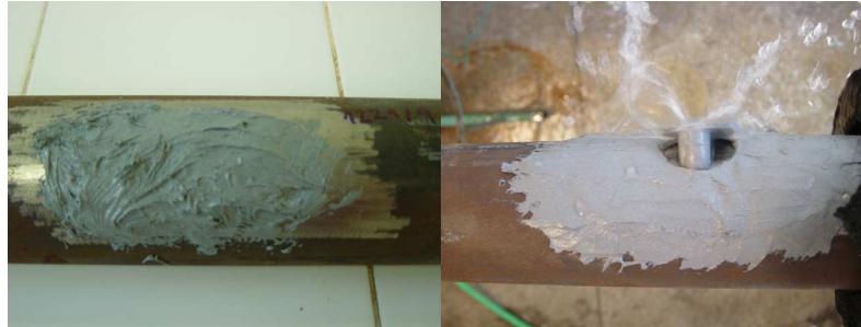
Figure 8: Epoxy Repair System B
