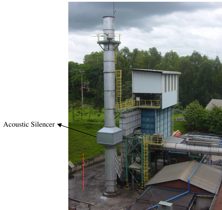
Figure 3. Noise silencer for exhaustion system
