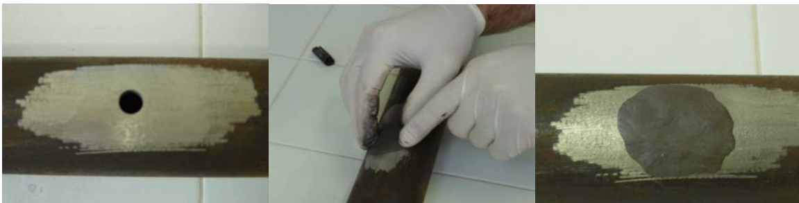
Figure 2 – Epoxy repair procedure
