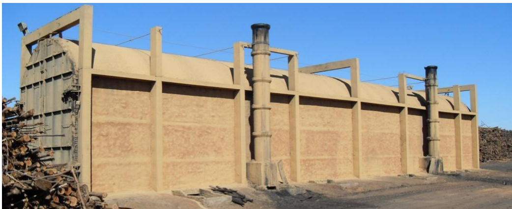
Figure 1. Rectangular masonry kiln: model RAC 220
