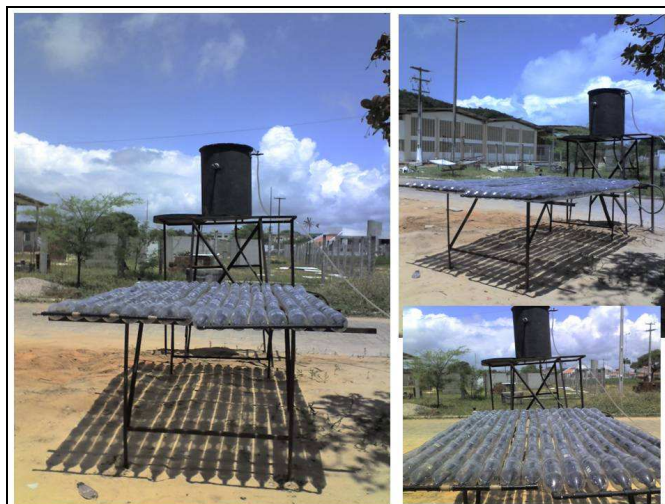
Figure 1. Solar heating system for disinfection of water.
