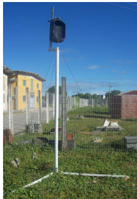
Figure 5. Absorber at the top of the tower
