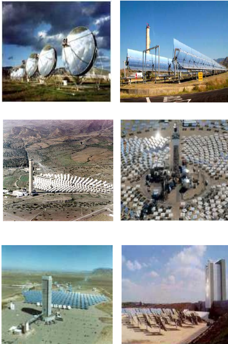
Figure 1. High-concentration, in operation.
