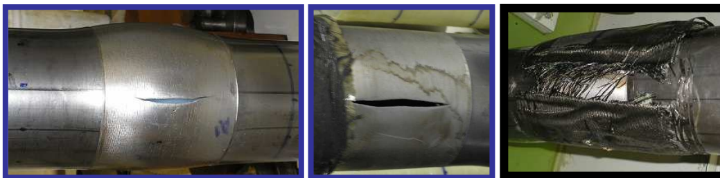
Figure 11. Place of the rupture in the steel pipe.
