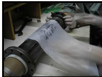
Figure 13. Preparing the Composite Repair.
