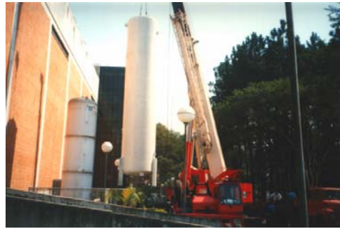
Figure 5. Installation of the new bigger cryogenic tank (26.000 litres).
